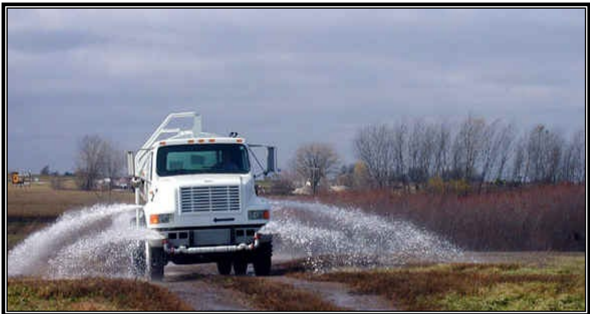
Figure IV - 4.21 Dust Suppression by Water Spray.
