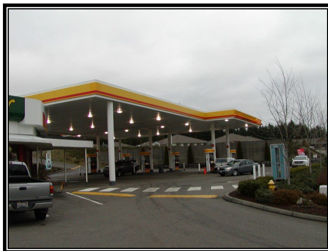
Figure IV - 5.3 Roof at Fueling Island to Prevent Stormwater Run-on.
