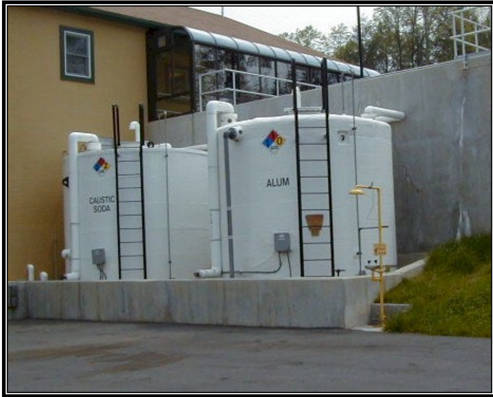
Figure IV - 4.19 Aboveground Storage Tanks with Secondary Containment.
