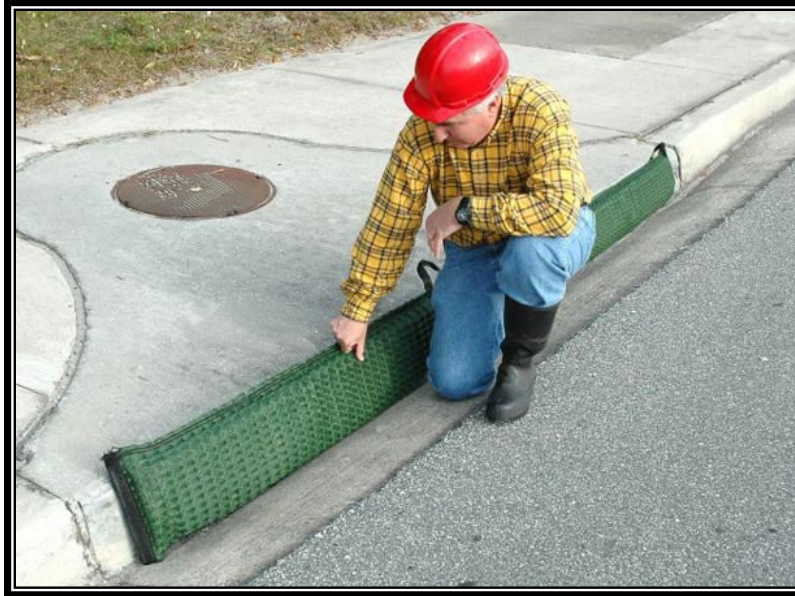
Figure IV - 4.20 Commercially Available Gutter Guard Being Replaced.
