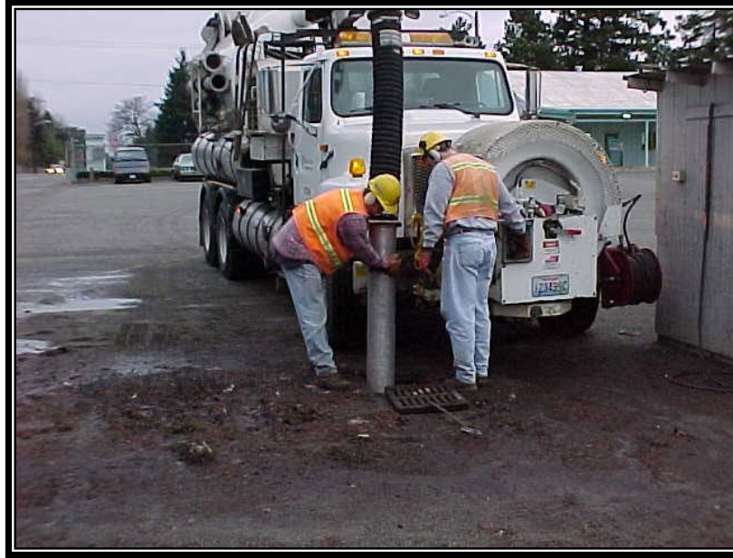
IV - Figure IV - 5.8 Catch Basin Cleaning with a Vacuum Truck.
