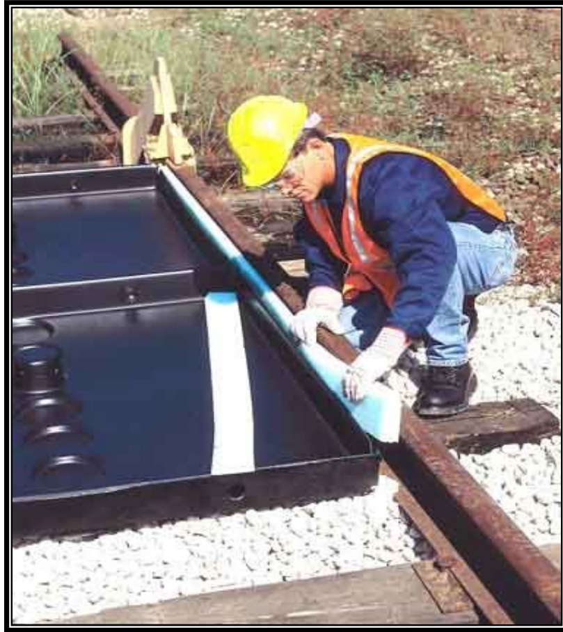
Figure IV - 4.4 Drip Pan for Connections at Loading and Unloading Areas for Liquid Material.
