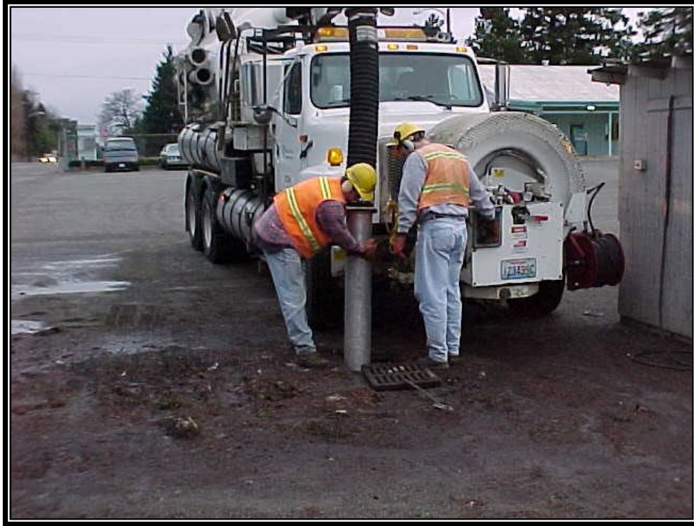
Figure IV - 4.23 Catch Basin Cleaning with a Vacuum Truck.
