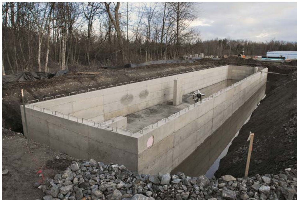
Wet vault construction at Bellingham
