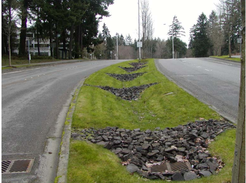
Biofiltration swale with check dams at Ecology headquarters
