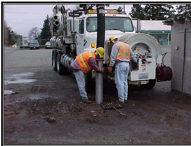
Figure 5.8. Catch Basin Cleaning with a Vacuum Truck.
