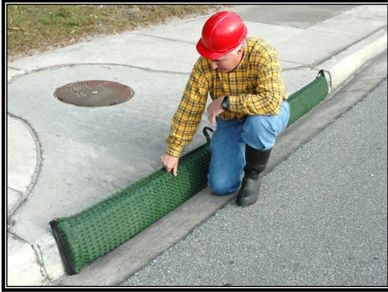
Figure 4.20. Commercially Available Gutter Guard Being Replaced.
