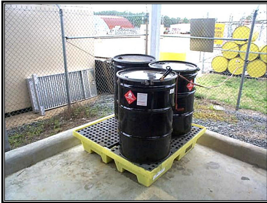
Figure 4.17. Temporary Secondary Containment.
