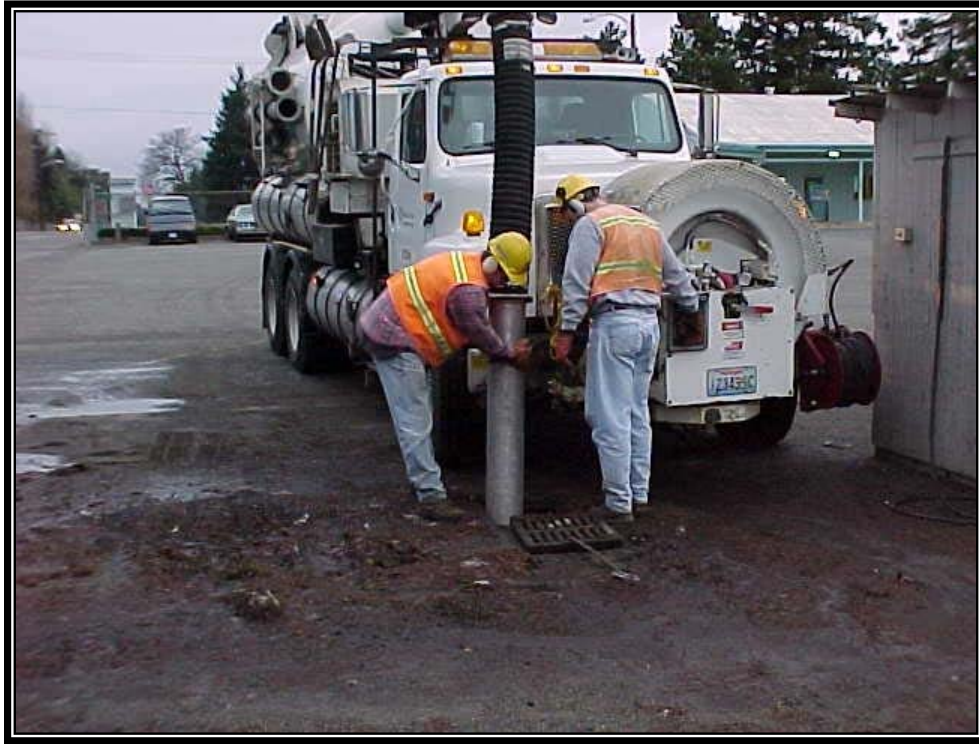
Figure 4.23. Catch Basin Cleaning with a Vacuum Truck.
