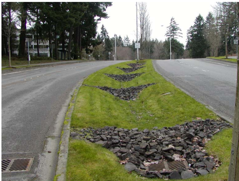
Biofiltration swale with check dams at Ecology headquarters
