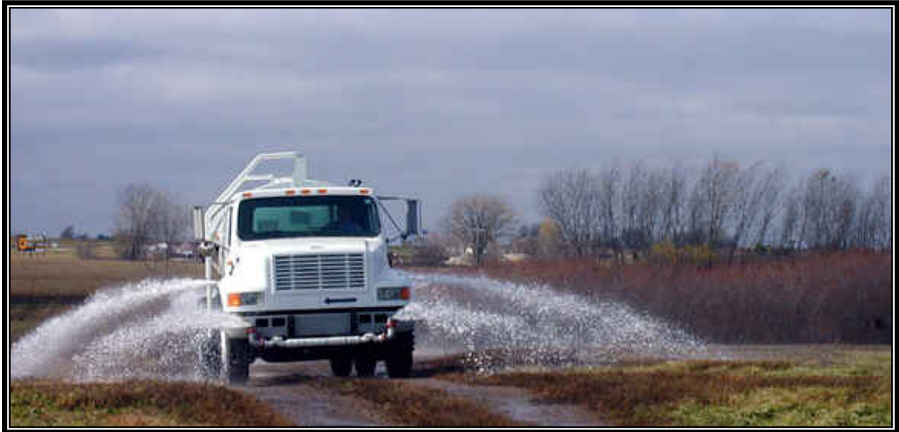
Figure 4.21. Dust Suppression by Water Spray.
