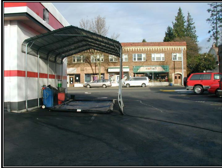
Figure 4.1. Wash Pad for Tool and Equipment Washing.
