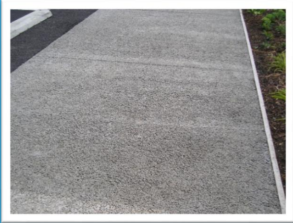
Porous asphalt uses a binding material to hold aggregate together
