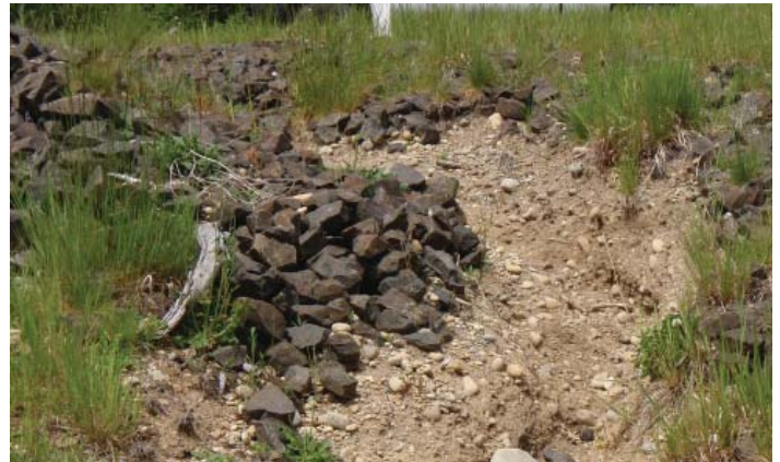
Erosion damages this dissipator.
