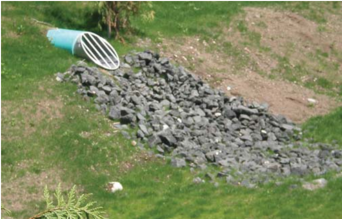
This energy dissipator is in good condition.
