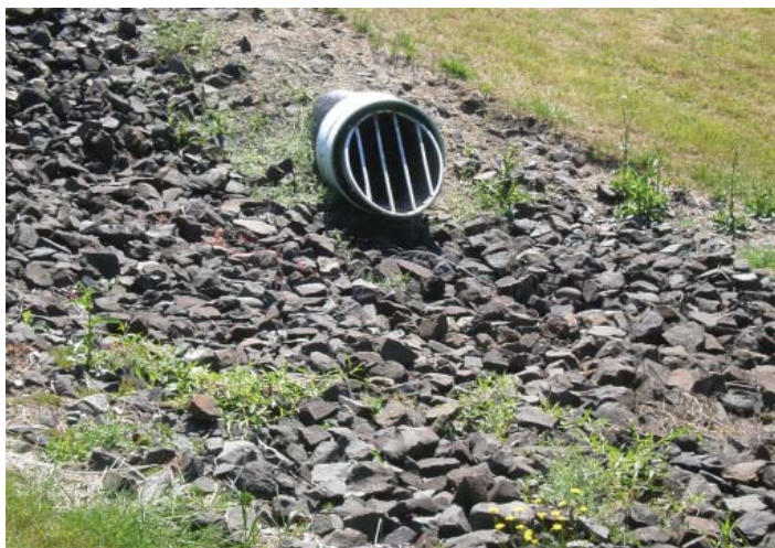
A well-maintained inlet pipe
