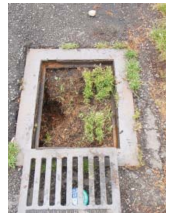
Catch basin clogged with sediment and debris
