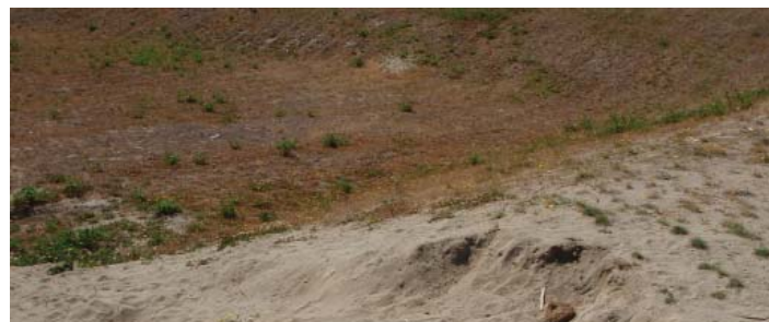
This berm is experiencing erosion.
