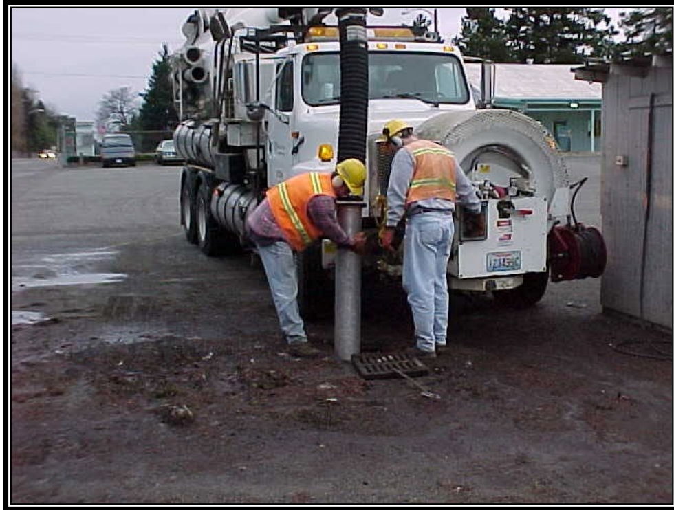
Figure IV - 4.23 Catch Basin Cleaning with a Vacuum Truck.
