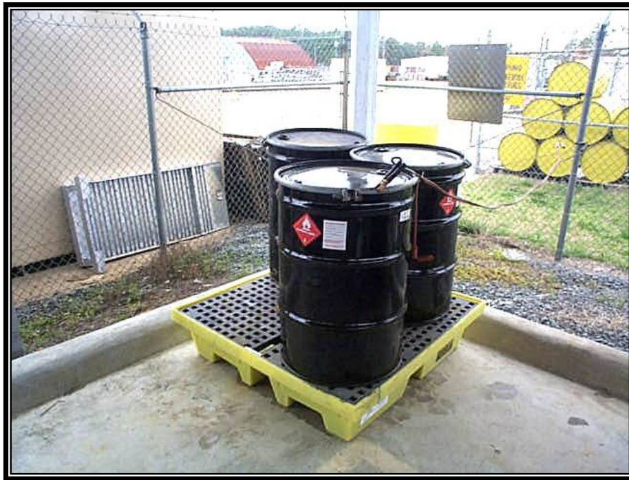
Figure IV - 4.17 Temporary Secondary Containment.
