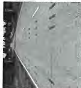
Completed Dowel Bar Retrofit (DBR) Project. Finished DBR project shows typical maintenance-free pavement in the old concrete pavement, strengthening the pavement and extending its life.
