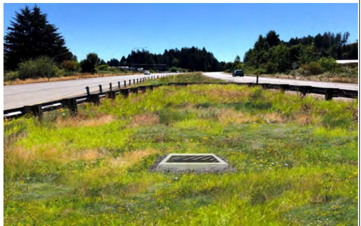
Biofiltration swale retrofit within US 101-27 median.
