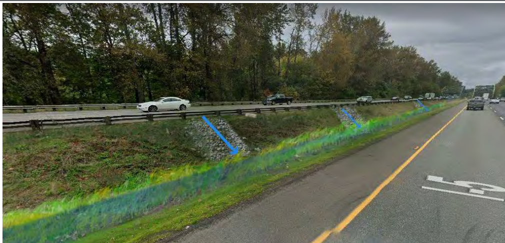
Biofiltration swale retrofit in WSDOT I-5 median, with additional curb cuts and erosion protection.
