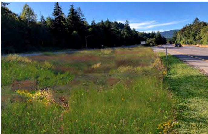
Biofiltration swale in SR 8 median.
