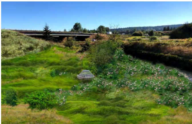
Constructed wetland retrofit between offramp and freeway. Overflow drain is piped back to existing storm main in median to eliminate a new outfall.
