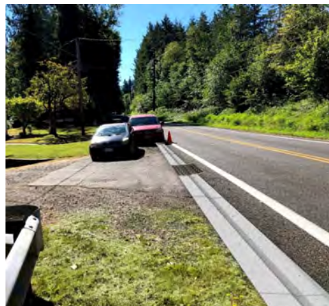
Site 1. New rolled curb and catch basin construction at 2330 Madrona Beach Rd.
