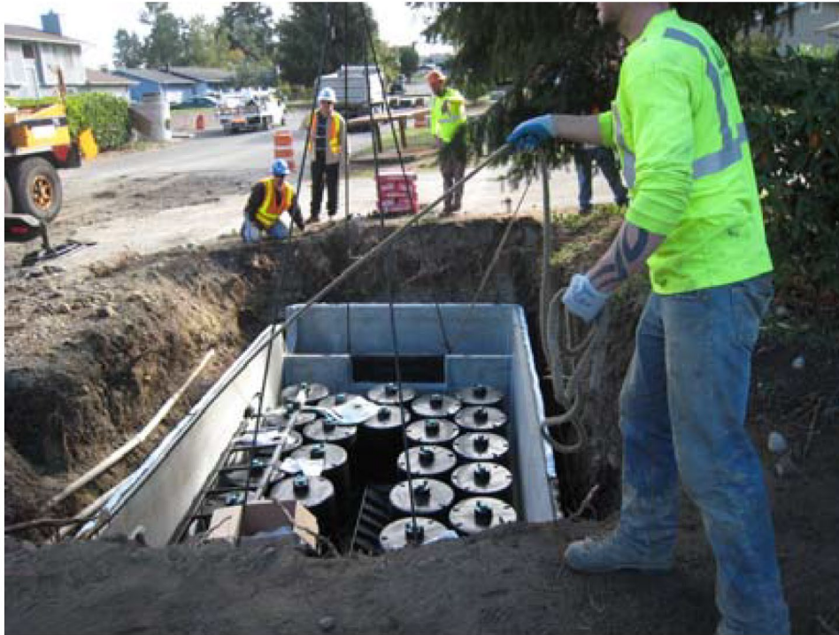
Stormfilter base unit in place
