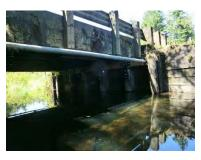
This bridge is located north of 140th Ave over Beaver Creek on Tilley Rd and was constructed in 1950. The bridge has a deteriorating timber pile substructure that requires frequent maintenance.
