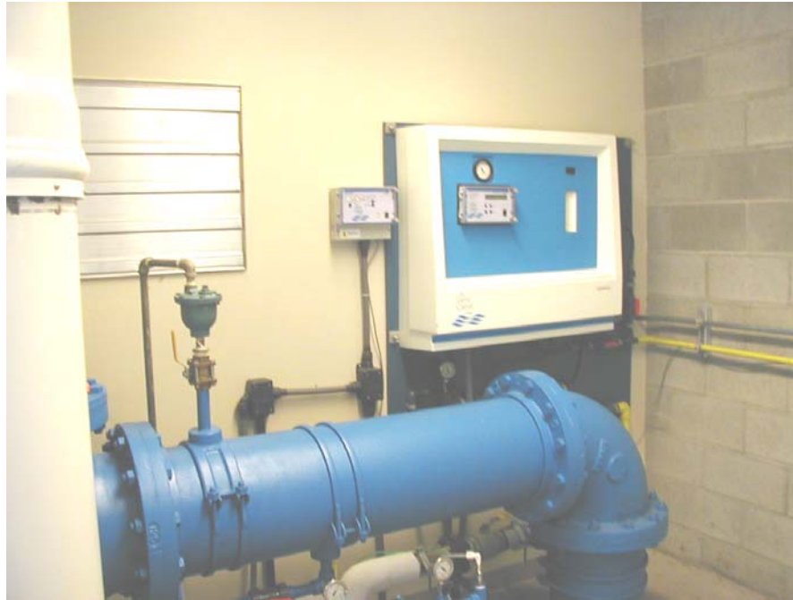
Figure 3-5 Photograph of the Chlorination Injection Equipment and Location
