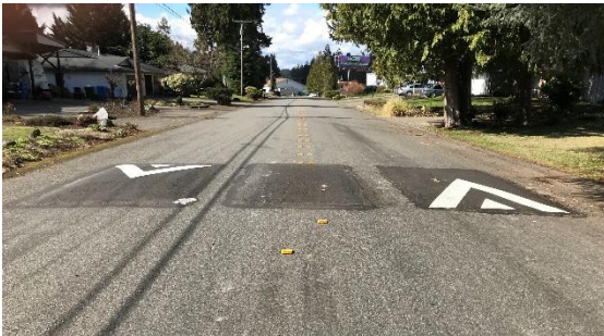
Location: Husky Way Install Date: July 2022 Device: Speed Cushions Cost: Approx. $15,000
