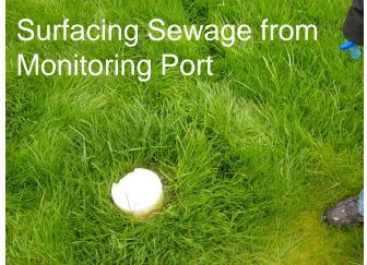
Deficiencies Noted: deficiencies must be corrected to ensure proper longevity of the Onsite Se
