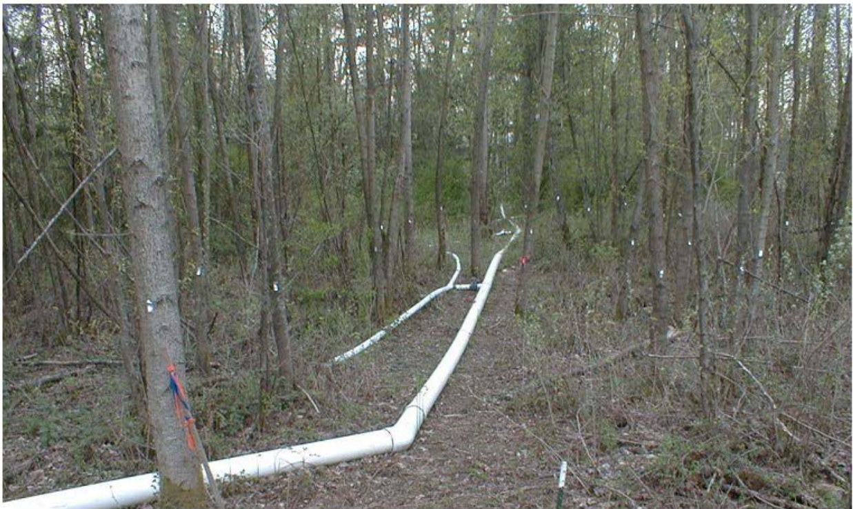
Figure 3-24. Manifold and Branches in wooded, vegetated spray field
