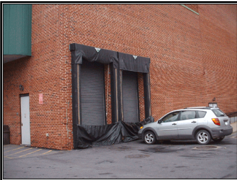
Figure 4.6. Door Skirts to Enclose the Trailer End of a Truck to Prevent Material Contact with Rainwater.
