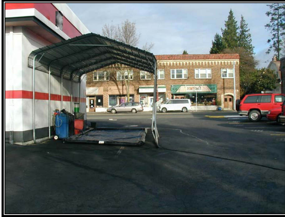
Figure 4.1. Wash Pad for Tool and Equipment Washing.
