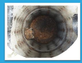
Well-functioning drywell with minimal sediment accumulation
