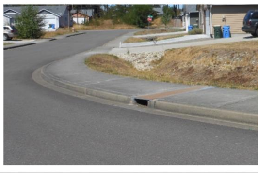
Sidewalk Underdrain, perspective
