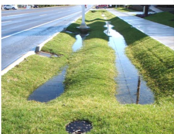
Thurston County curb cuts - conveying stormwater into a double swale
