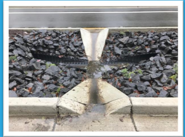
Thurston County Curb Cuts - moving stormwater into a culvert
