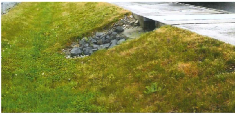
Sidewalk underdrain with an intact and clear splash pad at the outlet
