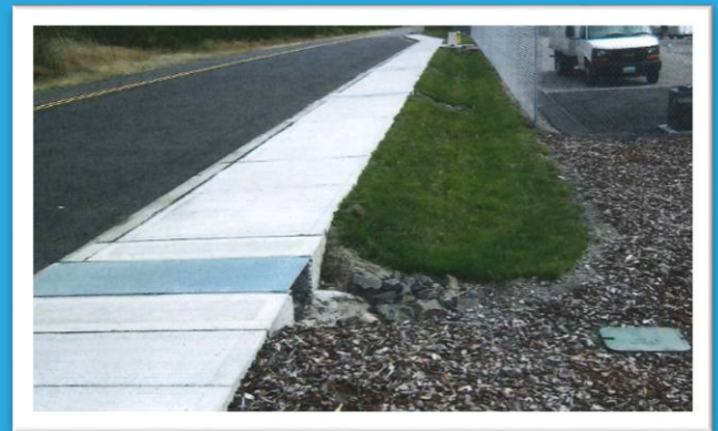
Sidewalk Underdrain with cement splash pad
