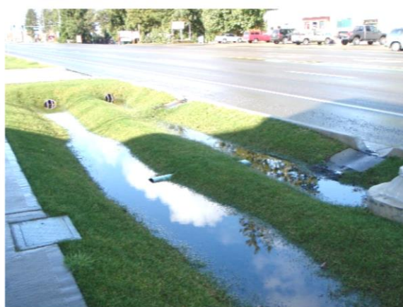
Thurston County curb cuts - conveying stormwater into a double swale
