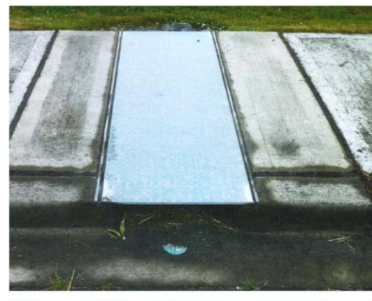
Sidewalk Underdrain, roadside inlet
