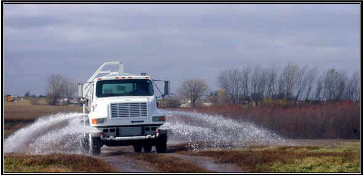
Figure 4.21. Dust Suppression by Water Spray.
