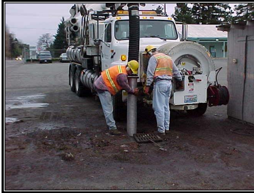
Figure 5.8. Catch Basin Cleaning with a Vacuum Truck.
