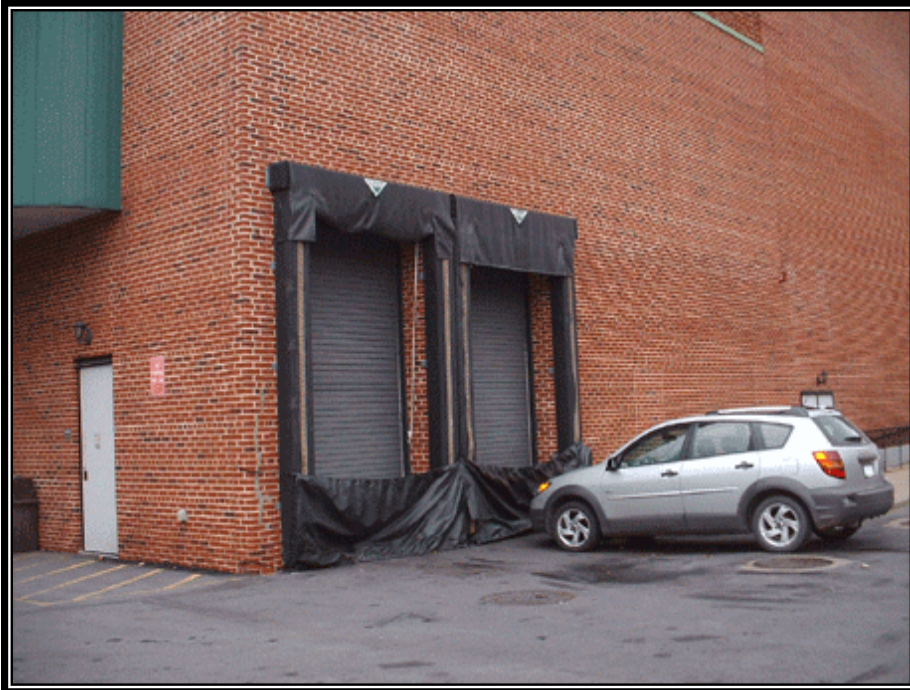
Figure 4.6. Door Skirts to Enclose the Trailer End of a Truck to Prevent Material Contact with Rainwater.
