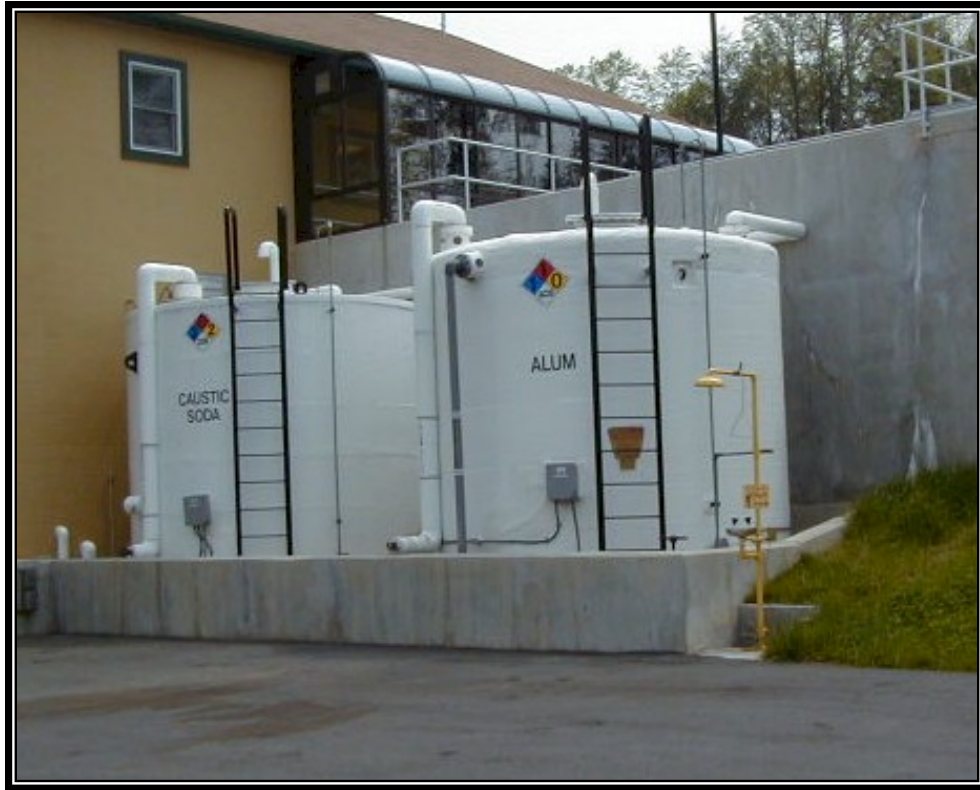
Figure 4.19. Aboveground Storage Tanks with Secondary Containment.
