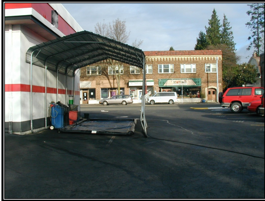
Figure 4.1. Wash Pad for Tool and Equipment Washing.
