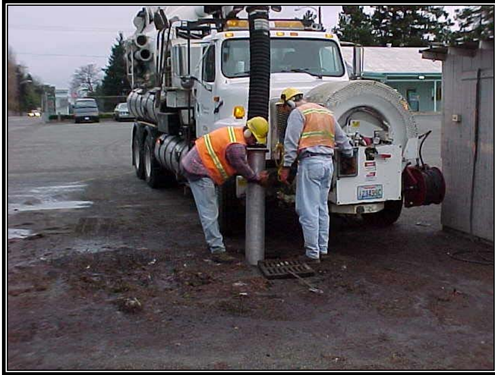
Figure 4.23. Catch Basin Cleaning with a Vacuum Truck.
