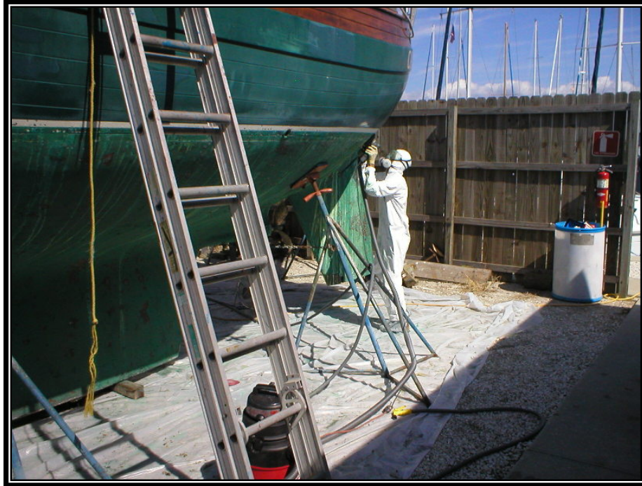
Figure 4.22. Drop Cloth Used During Hull Sanding.
