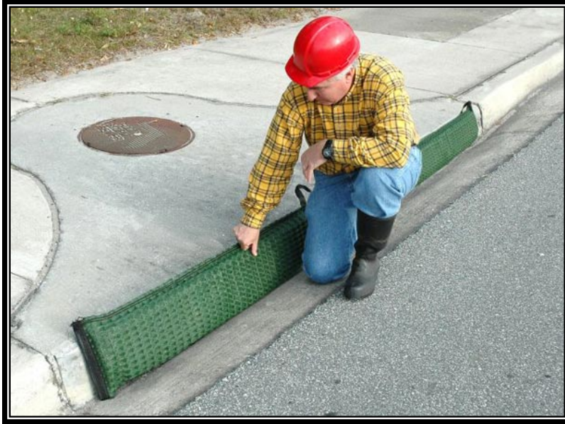
Figure 4.20. Commercially Available Gutter Guard Being Replaced.
