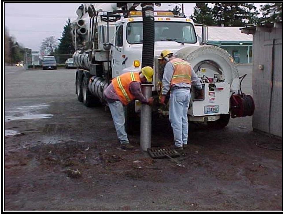
Figure 4.23. Catch Basin Cleaning with a Vacuum Truck.
