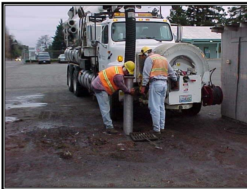
Figure 5.8. Catch Basin Cleaning with a Vacuum Truck.
