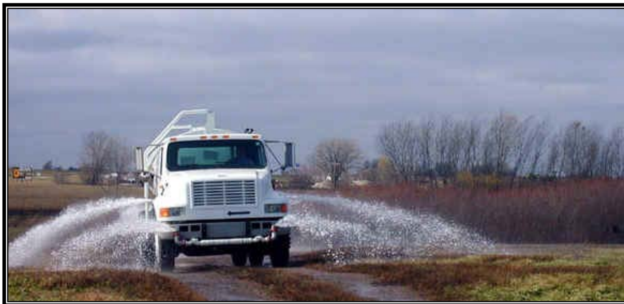
Figure 4.21. Dust Suppression by Water Spray.
