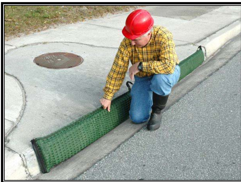
Figure 4.20. Commercially Available Gutter Guard Being Replaced.
