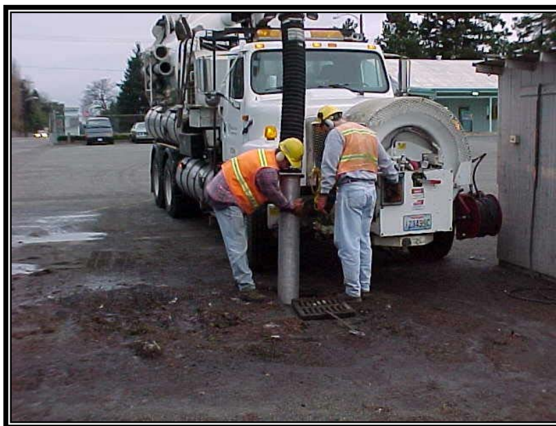
Figure 5.8. Catch Basin Cleaning with a Vacuum Truck.
