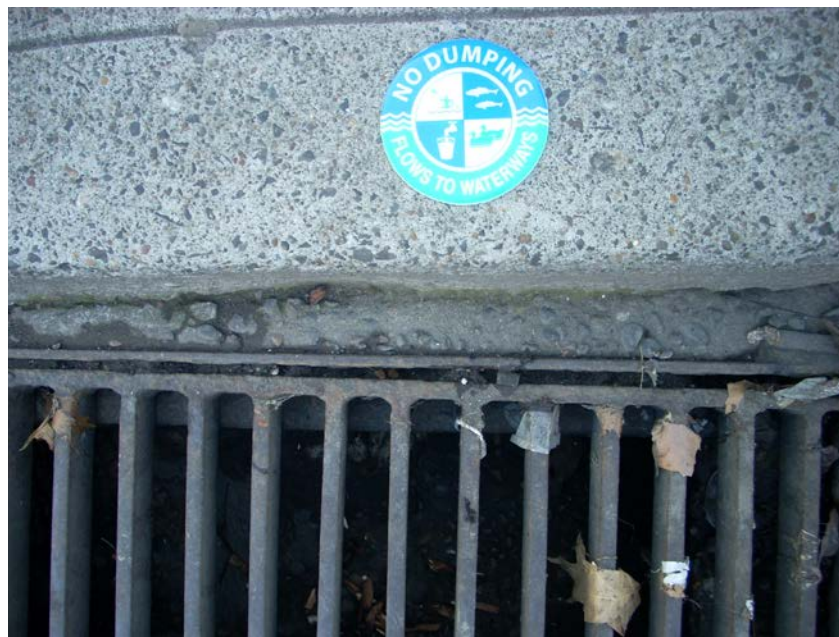
Figure 4.24. “No Dumping” Storm Drain Button.
