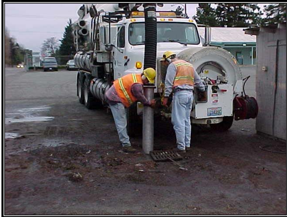
Figure 4.23. Catch Basin Cleaning with a Vacuum Truck.
