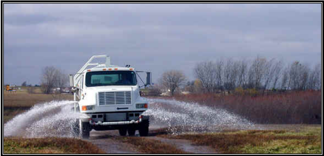
Figure 4.21. Dust Suppression by Water Spray.
