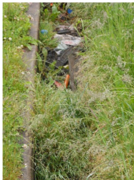
This level spreader is clogged with garbage and weeds
