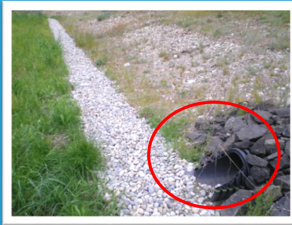
Dispersion devices can be made of small rocks or concrete and are often fed by stormwater pipes
