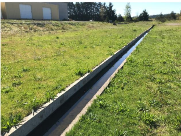
This level spreader is clean and clear – in great condition
