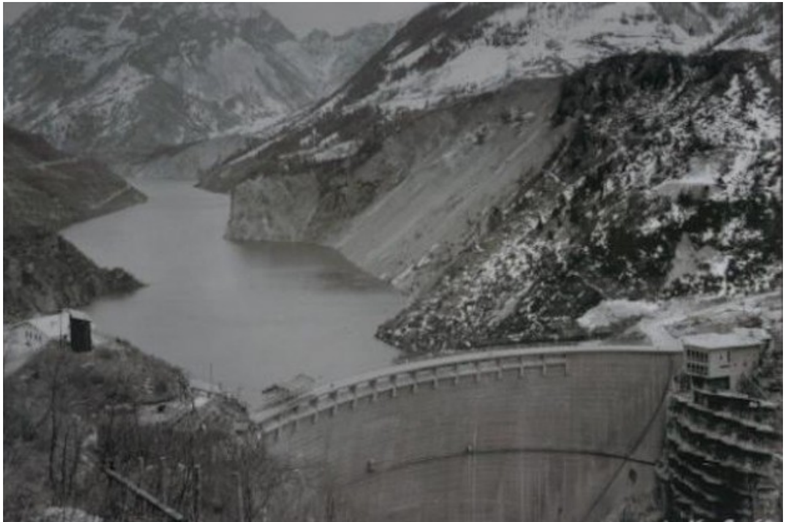
Type 4. Seiche Generated by Large Landslide impacting Lake with a 400 meter high dam (Italy)
