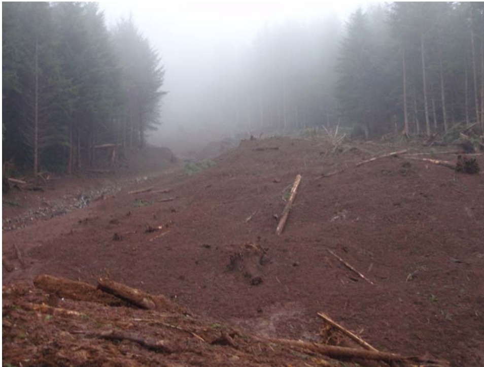
January 2009 - Middle Portion of the slide (900-1200') Looking upslope the path of the slide debris is apparent and the transition to debris flow/torrent has occurred. The forest has been leveled in the path of the debris
