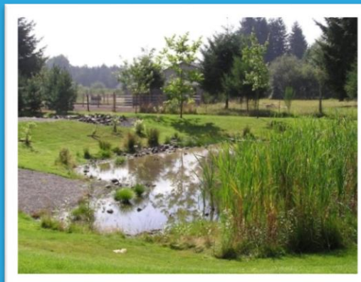
Figure 1: Wet Pond Typically holds water year-round
