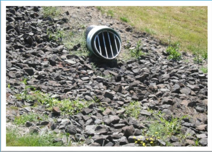
A well-maintained inlet pipe and "riprap" splash pad
