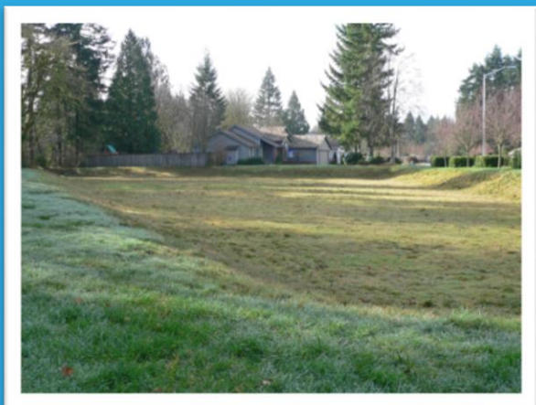
Figure 2: Dry Pond Designed to function as an open field until the rainy season
