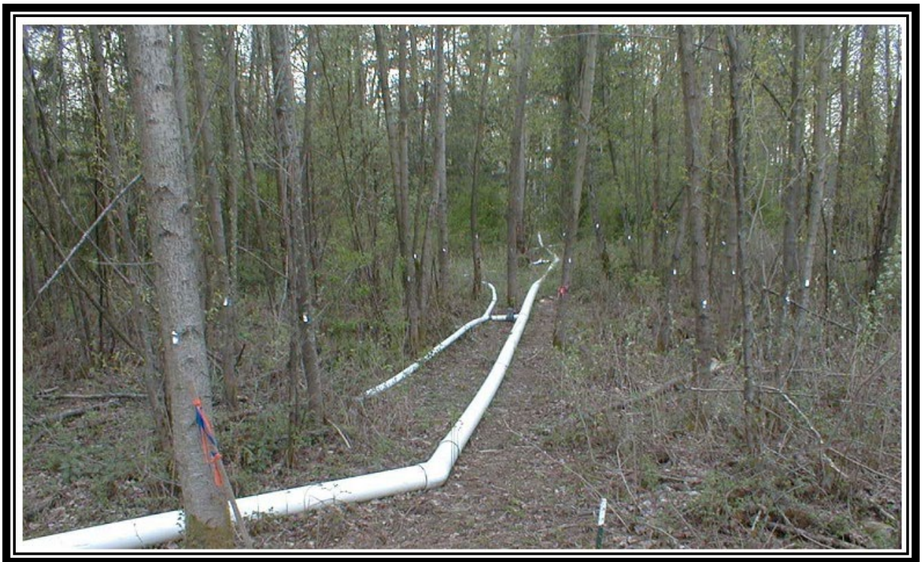
Figure II – 3.22 Manifold and Branches in wooded, vegetated spray field
