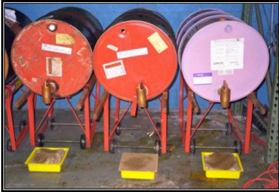
Figure IV - 4.18 Mounted Containers with Drip Pans.
