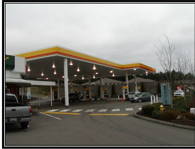
Figure IV - 4.7 Roof at Fueling Island to Prevent Stormwater Run-on.
