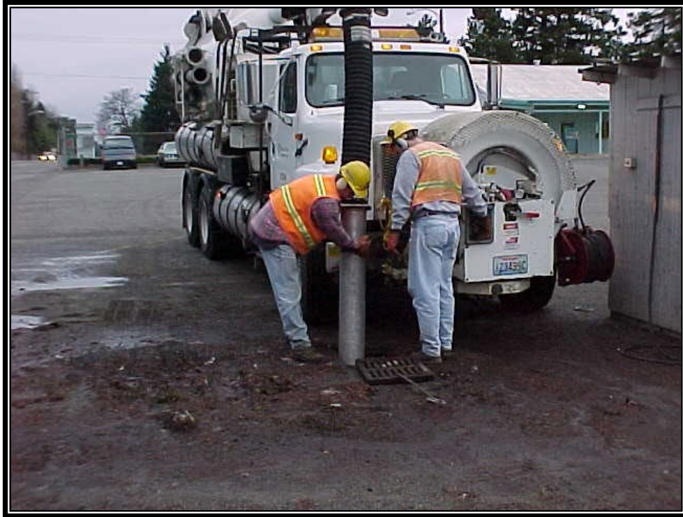
Figure IV - 4.23 Catch Basin Cleaning with a Vacuum Truck.
