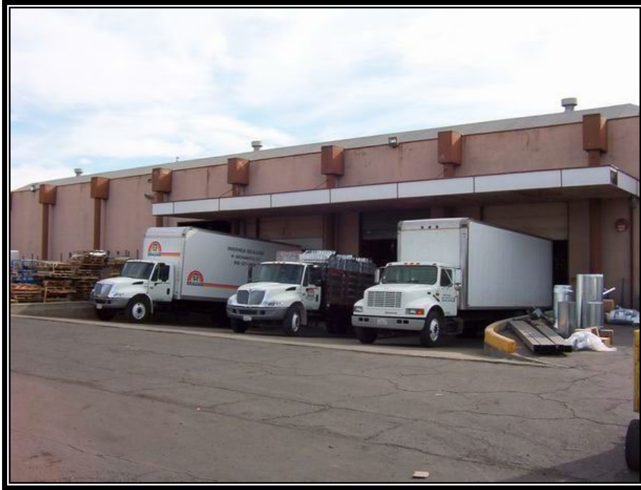
Figure IV - 4.5 Loading Docks with an Overhang to Prevent Material Contact with Rainwater.
