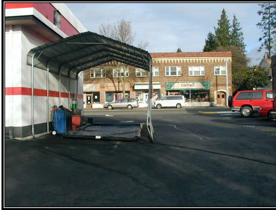
Figure IV - 4.1 Wash Pad for Tool and Equipment Washing.
