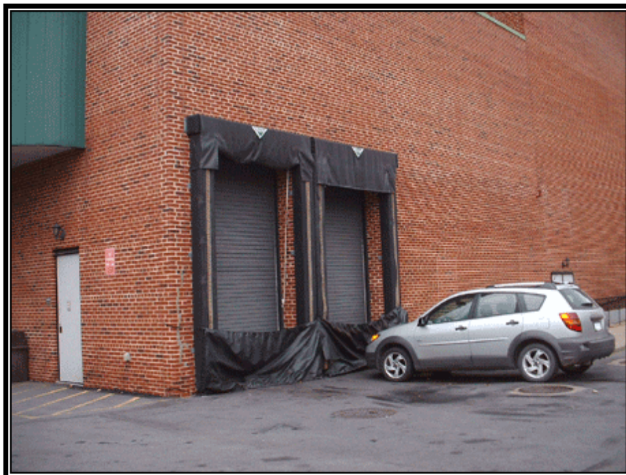
Figure IV - 4.6 Door Skirts to Enclose the Trailer End of a Truck to Prevent Material Contact with Rainwater.
