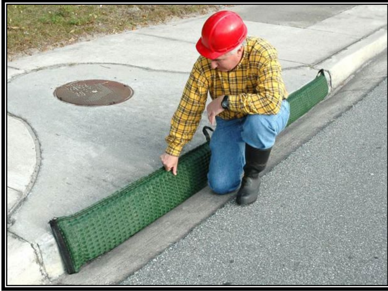
Figure IV - 4.20 Commercially Available Gutter Guard Being Replaced.
