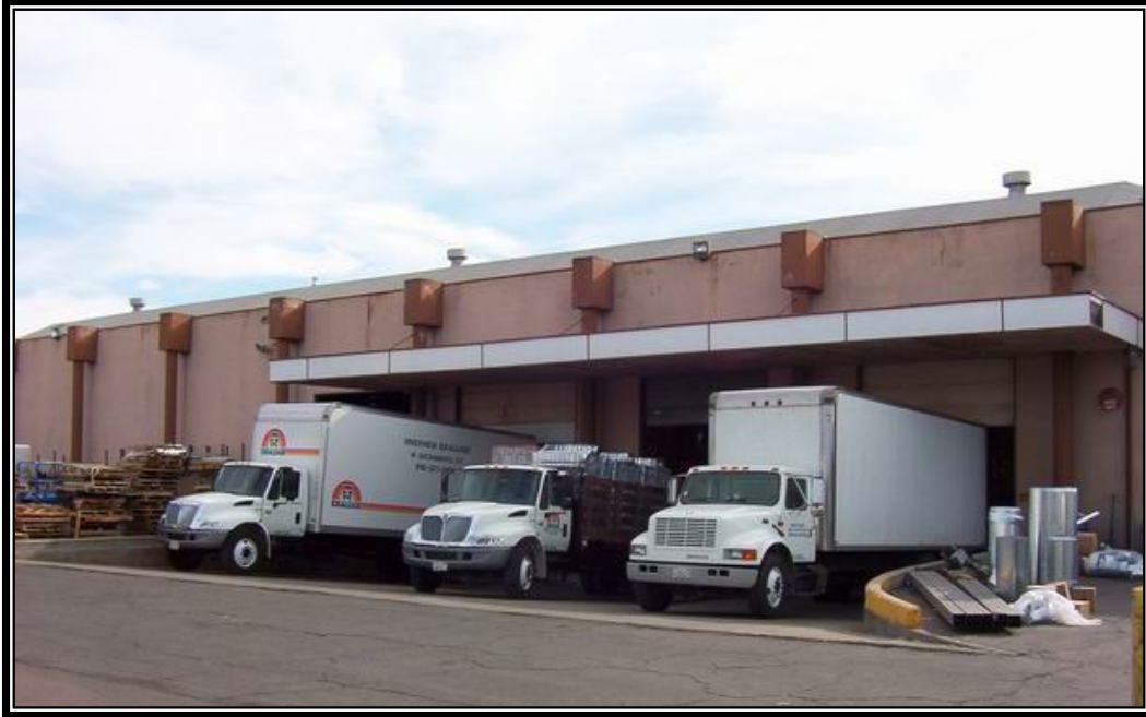
Figure IV - 5.2 Loading Docks with an Overhang to Prevent Material Contact with Rainwater.
