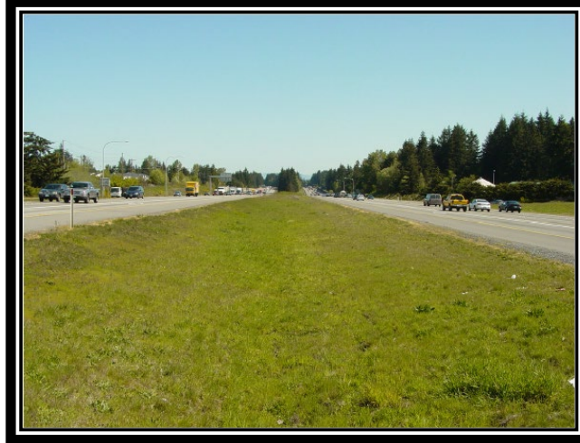
Vegetated Filter Strip in Median Along I-5 in Snohomish County
