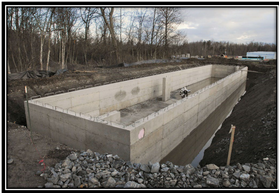
Wet vault construction at Bellingham
