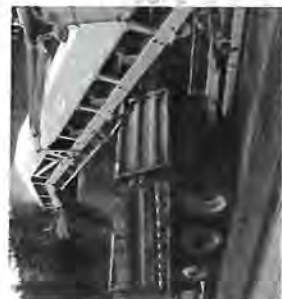
Millage operation, removing worn asphalt wearing surface and the top two inches of the base course are removed, leaving the rest of the pavement intact.
