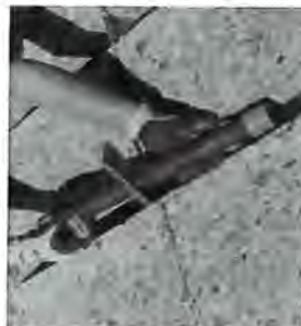
A worker installs dowel bars into a slot on a Dowel Bar Retrofit project. The dowel bars transfer heavy truck loads from panel to panel.
