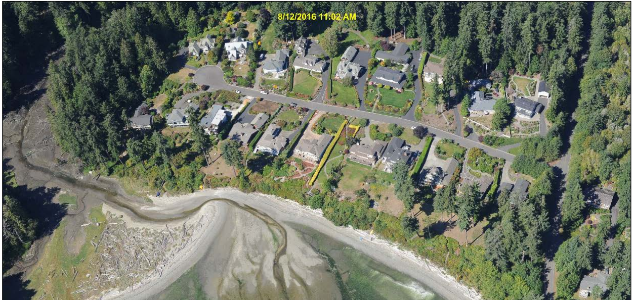
Figure 9: Construction of a single-family home by an owner, lessee, or contract purchaser for their own use or for the use of their family is exempt from the requirement for a substantial development permit. However, a variance or conditional use permit may be required. (Washington Coastal Atlas photo.)
