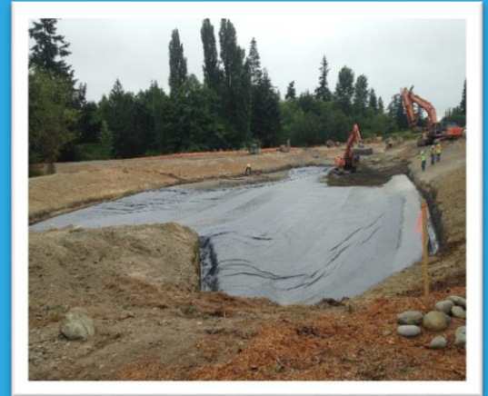
Source: Kitsap County Constructed Wetland – during construction
