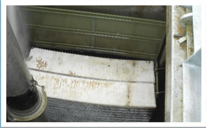
Oil/Water Separator after cleaned
